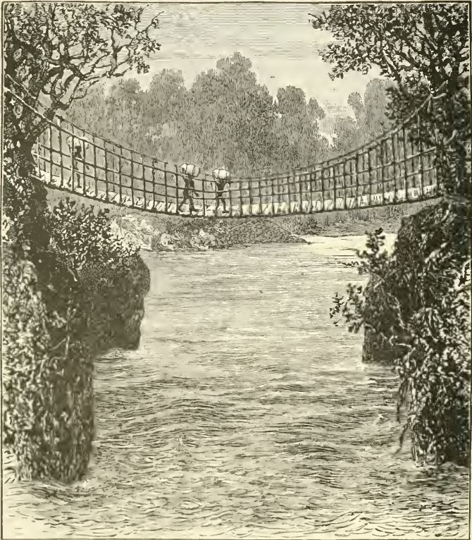
SUSPENSION BRIDGE ACROSS THE E. ITURI.
